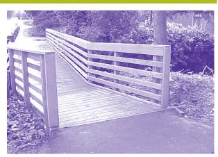
The existing two-lane bridge did not include a walkway. Rather than replacing the bridge, which would have been very expensive, county engineering staff came up with a cantilevered design, hanging the ped bridge onto the existing structure.
