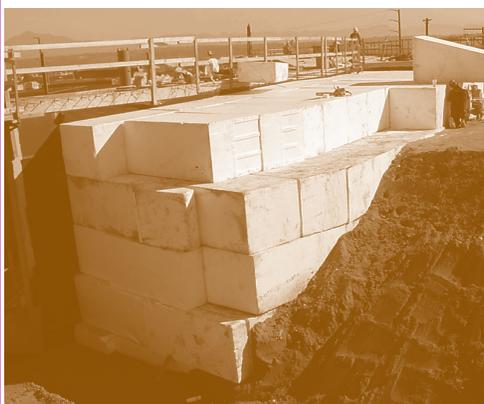
Since the underlying ground was soft, normal earth fill would have caused the roadway to settle and side slopes to possibly fail. Using geofoam we raised the roadway and built taller abutments without adding any weight and thus had no settlement problem. Susbauer Bridge was successfully completed in 2007.
